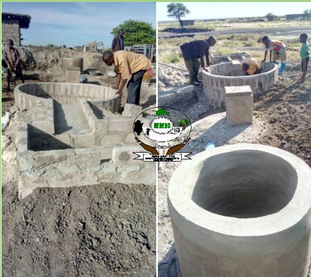
Photo 64: Biogas construction progress at Inolelo Village
