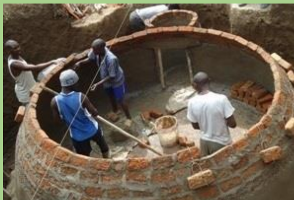
Photo 24: Construction of fixed Chinese dome
