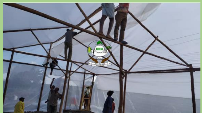
Photo 47: Group members participating in construction of Greenhouse at Ngundangali village
