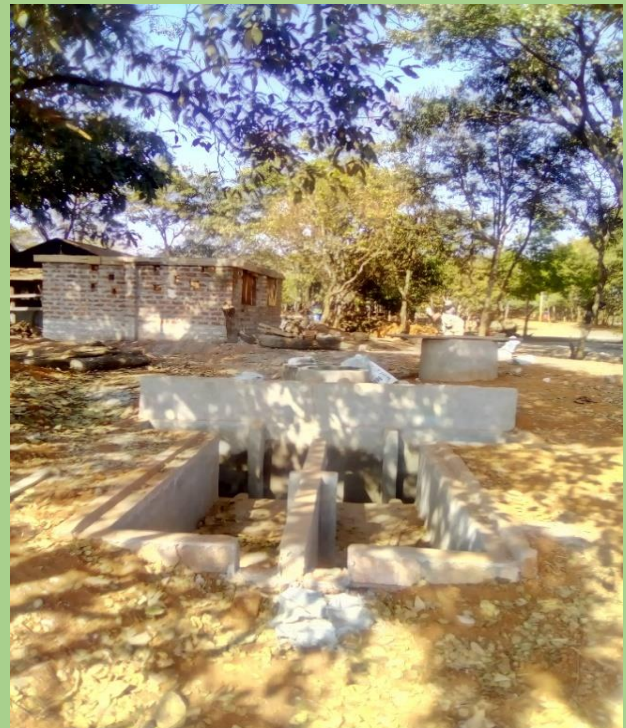
Photo 26: On right picture showing immersed fixed dome, cow dung mixing chamber, outlet slurry channels and new constructed kitchen at lintel stage, back to the new constructed kitchen seen old kitchen used by the school to cook meals for pupils using firewood.
