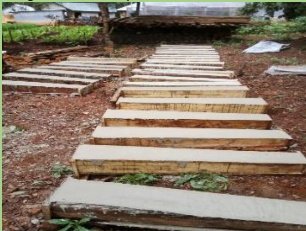
Photo 14: Beacons fabrication in process for demarcating rivers and water sources shared by the host and refugee's community.
