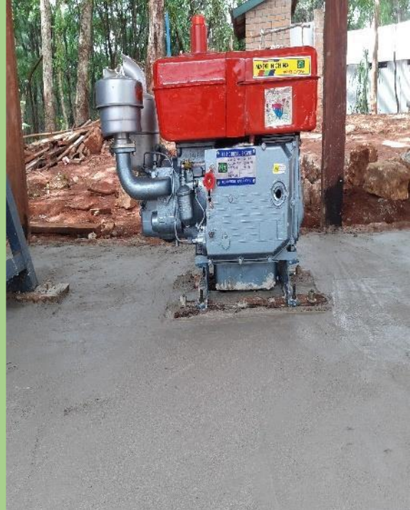
Photo 30: Installed engine at Nduta camp
