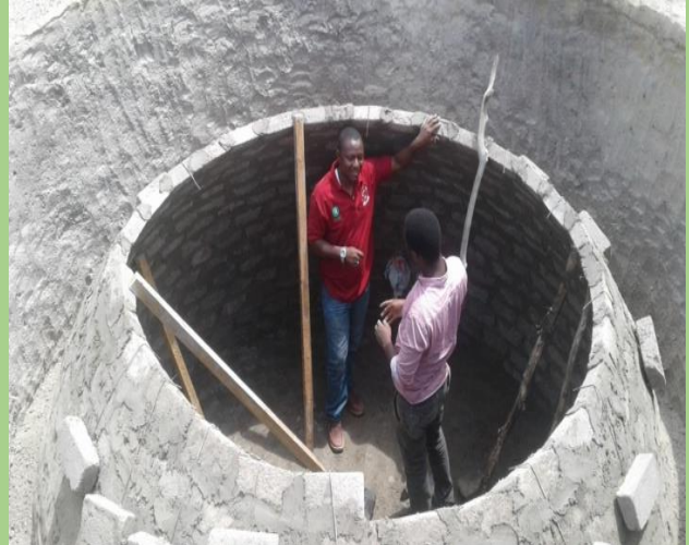
Photo 68: Mr. Enock Makinda from CAMATEC (first at left) discussing with one of the REDESO's Officer in the Biogas DIGESTER during the construction at Nhobola Village.
