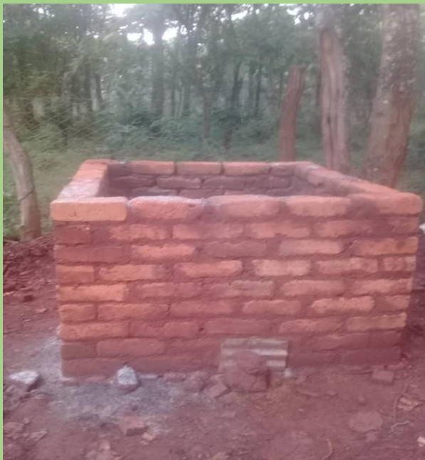
Photo 36: Constructed brick kiln in Nduta Camp
