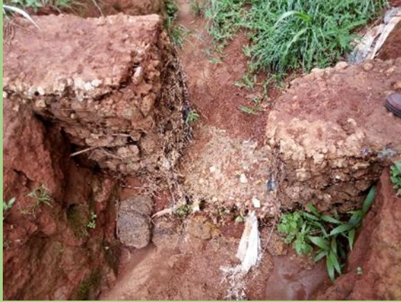
Photo 16: Gabion showing a healing process of a gully at Nduta camp in Kibondo.
