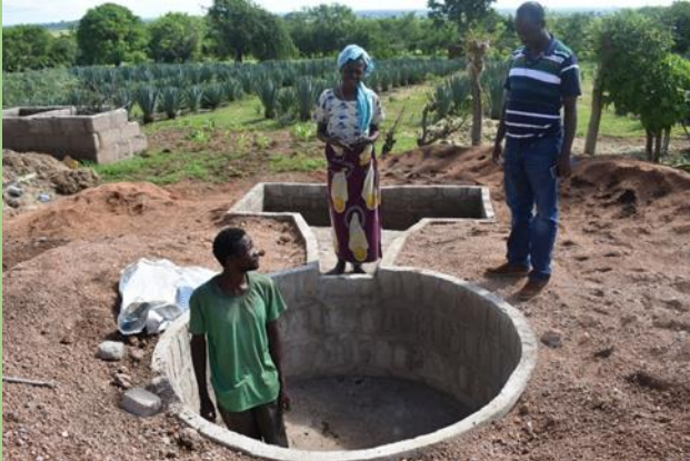
Photo 66: REDESO Project Coordinator (Charles Buregeya at right hand side) with Suzana Philipo and her son (in the outlet chamber) having a progress checking up of the Biogas structure during final process of construction at Nhobola village.
