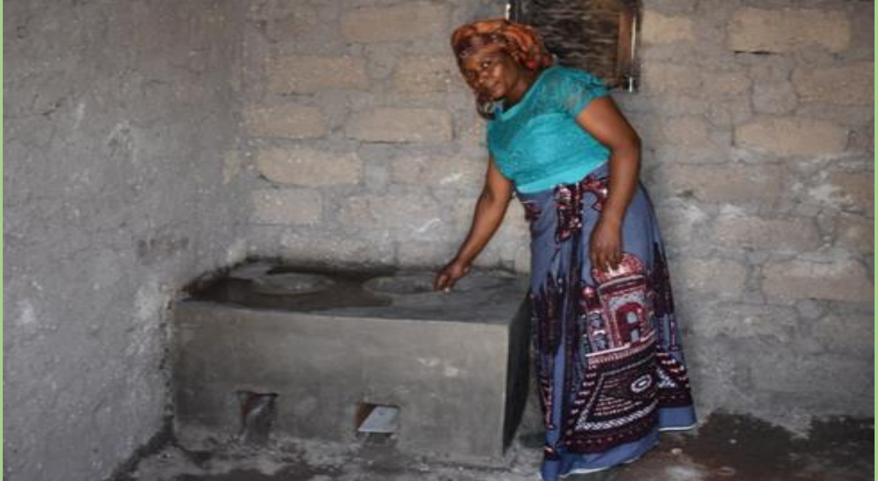
Photo 83: One of the Cooking stoves constructed at Inolelo village.
